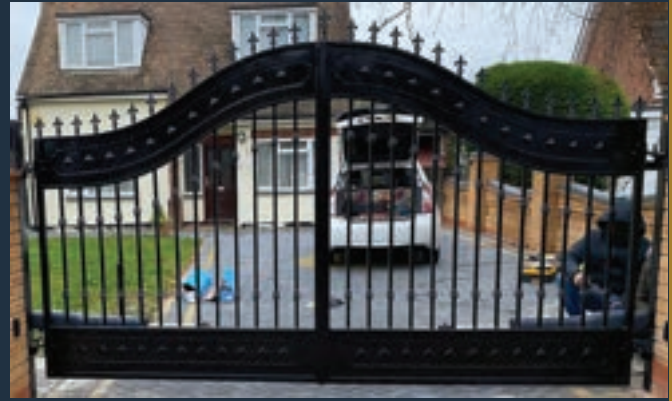
GATE- ELM 02 , Swing Gate
