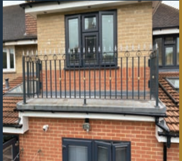
ELM 15, Balustrade Railing
