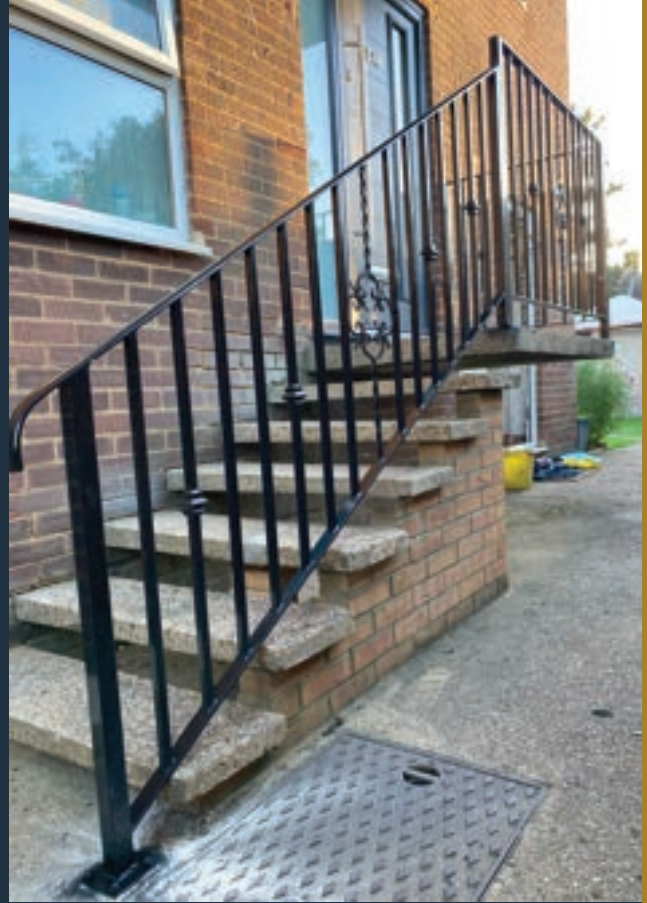
ELM 19, Stair Balustrade Railing
