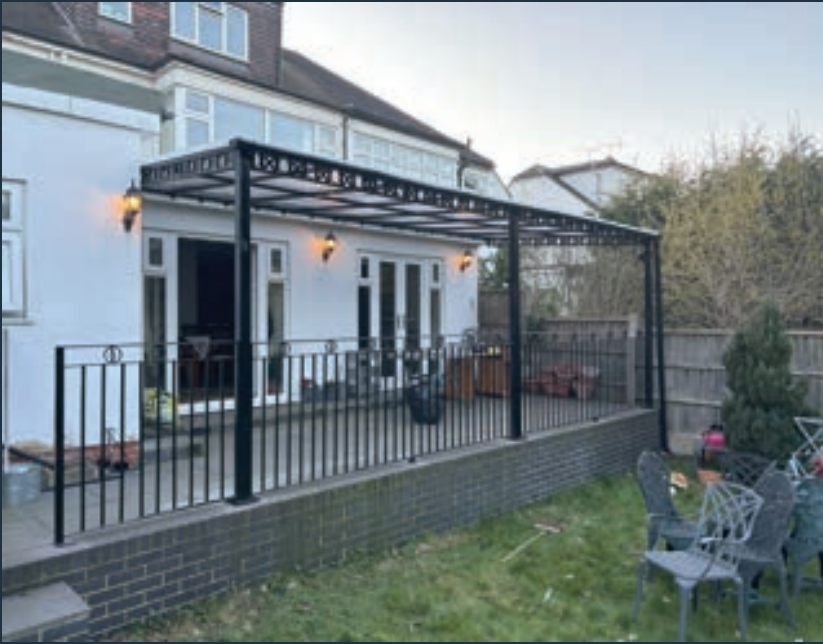
ELM 12, Railing & Pergola
