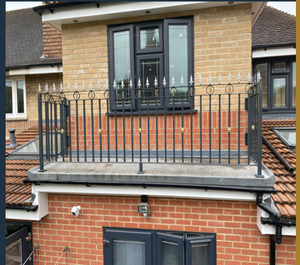
ELM 15, Balustrade Railing
