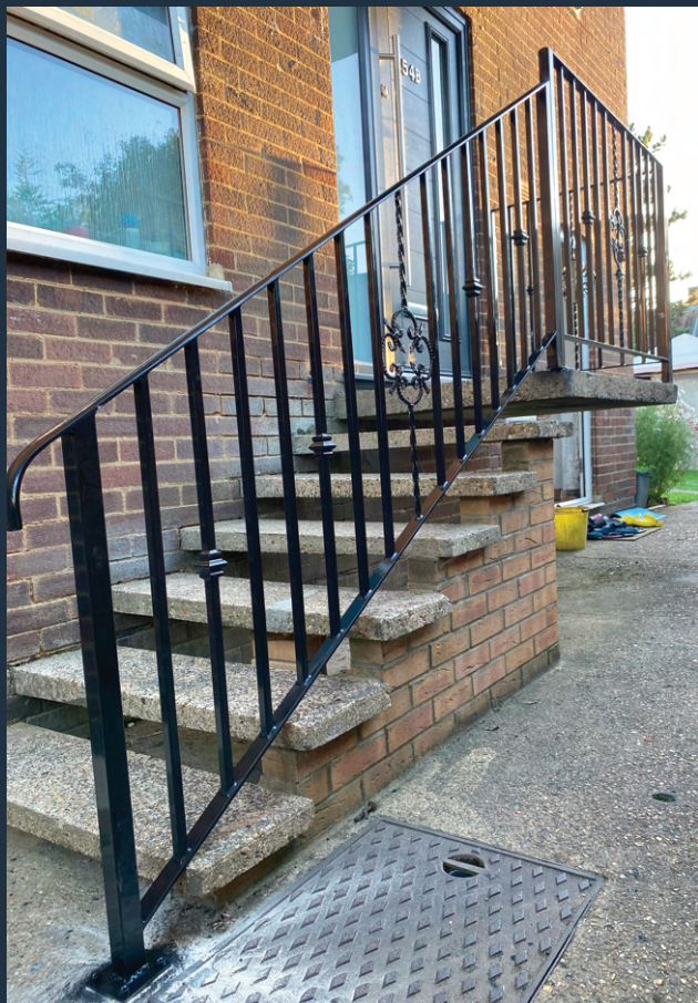
ELM 19, Stair Balustrade Railing
